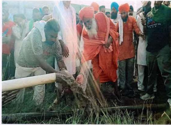
Plate-3: Photograph showing water being abstracted from the tubewell installed in the parking area
